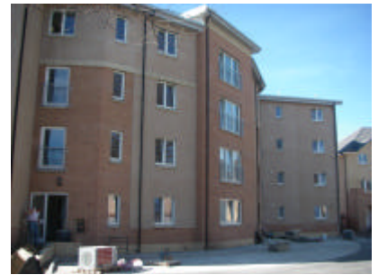
The City Hospital site nearing completion in late 2007.
