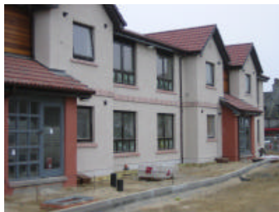
Merrivale, Dyce under construction.
