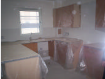
Work in progress at Portland Street, Aberdeen
