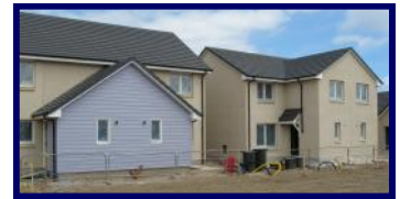
Shared equity houses in progress at Portlethen.
