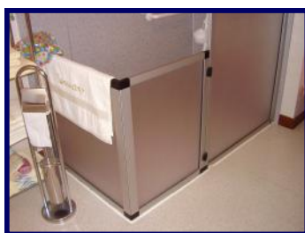
Adaptation completed by Care & Repair
