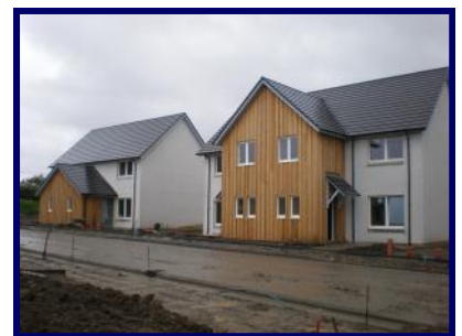
The Mintlaw site nearing completion in late 2008.
