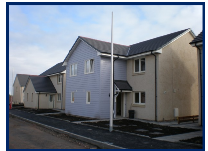
The Portlethen site nearing completion in late 2009.
