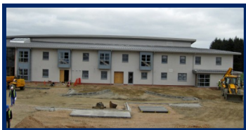
Very sheltered scheme at Abbey Court, Mintlaw nearing completion in April 2010
