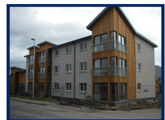
General needs scheme at Arran Avenue, Aberdeen under construction in August 2010.
