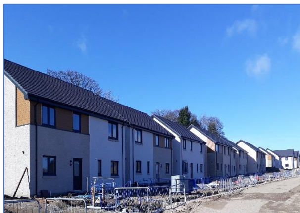
Maidencraig, Aberdeen, under construction 2019
