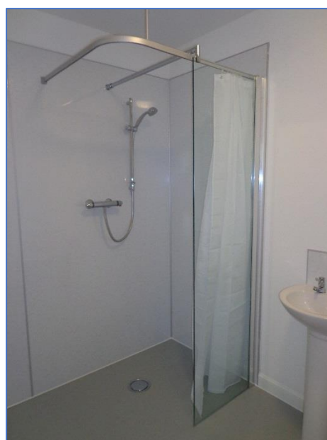
Wet floor shower adaptation by Castlehill.
